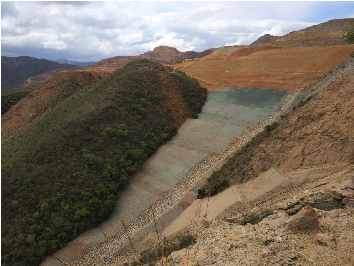
The south waste rock pile at the Thio mine rehabilitated and in the process of revegetation.
