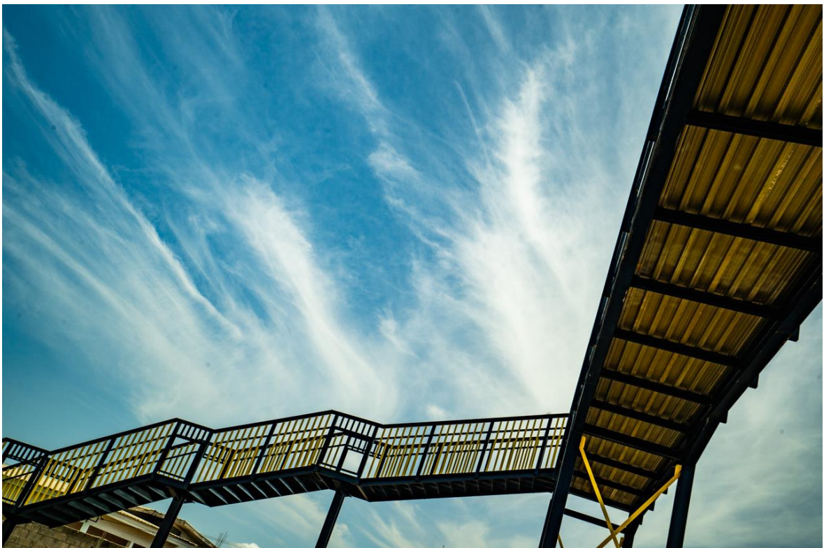
One of the six pedestrian footbridges constructed by Setrag for safe passage over the railway.
