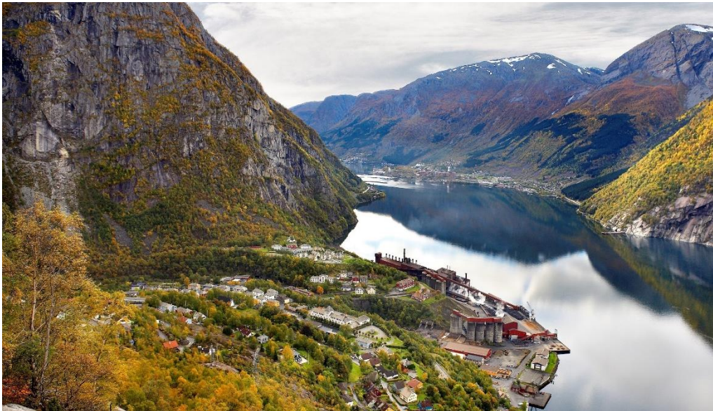
Tyssedal, Norway : The TTI conversion plant produces titanium dioxide slag and high purity cast iron from ilmenite
